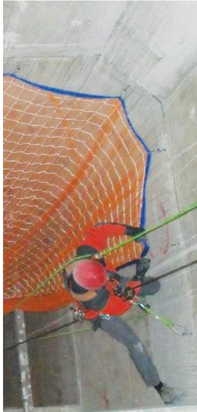
SAFETY NET APPLICATION FOR ELEVATOR SHAFT
