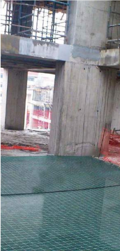
SAFETY NET APPLICATION FOR WIDE FLOOR OPENINGS
