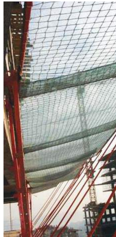
SAFETY NET PLATFORM APPLICATIONS FOR FACADES
