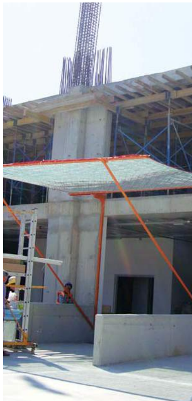
SAFETY NET APPLICATION FOR BUILDING ENTRANCES
